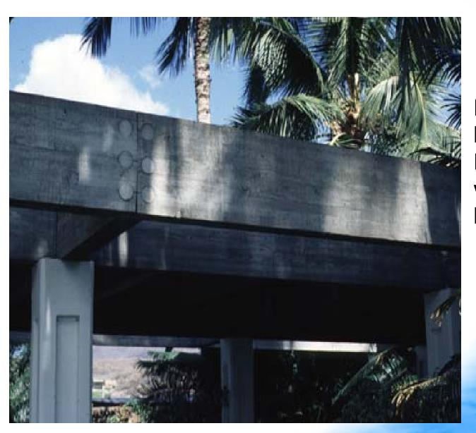
Exterior and Interior Glulam Beams Treated with Tribucide II™
